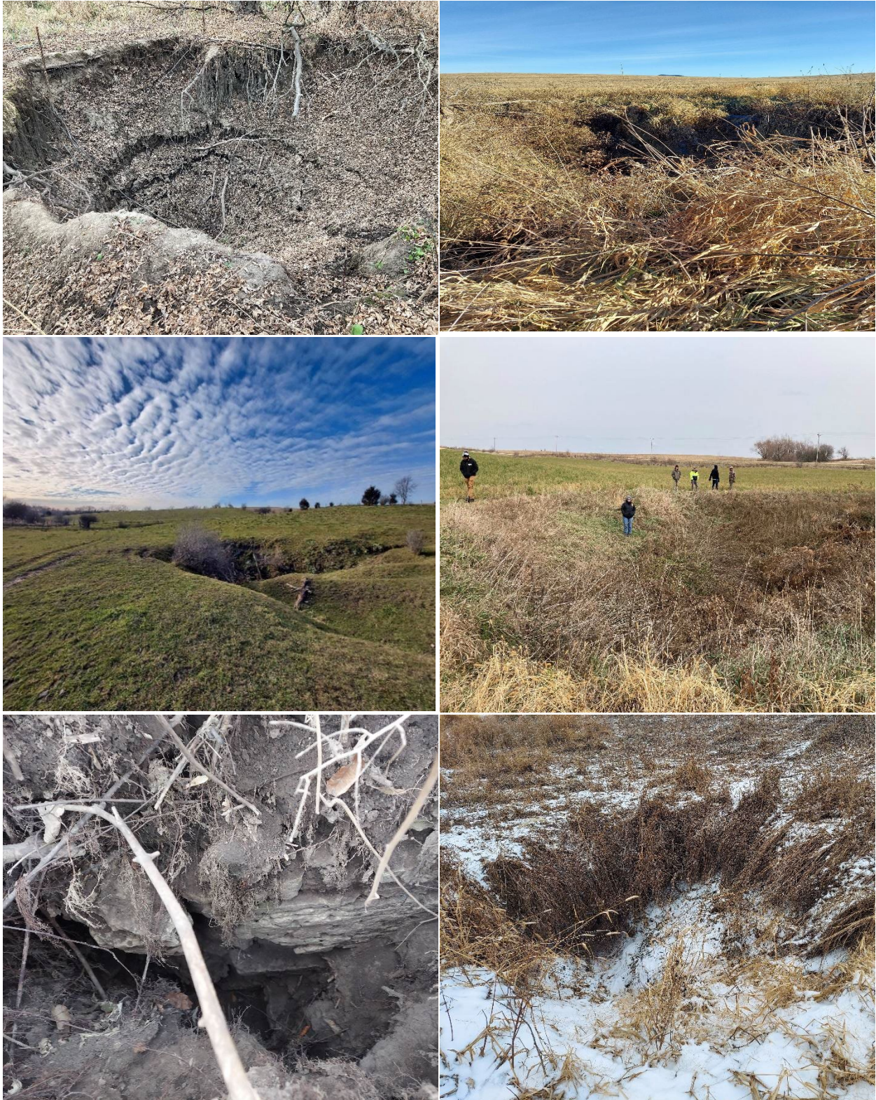
Figure 20. Example sinkholes found in the Trout Run Watershed. Top left: Newly formed sinkhole in Trout Run. Top right: Sinkhole receiving tile discharge and overland flow from cropland. Middle left: sinkhole in
