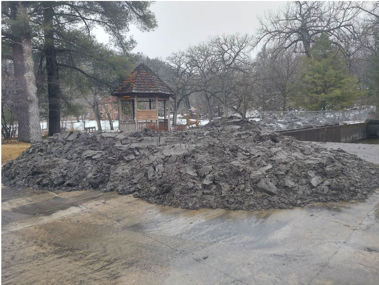
Figure 9. 303.13 tons of sediment accumulated in the Chuck Gipp Decorah Fish Hatchery clarifiers from five rainfall events in July and August 2022.
